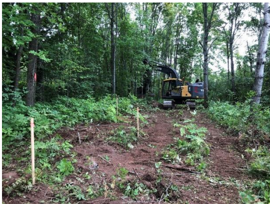
Clearing the new stream corridor area.
