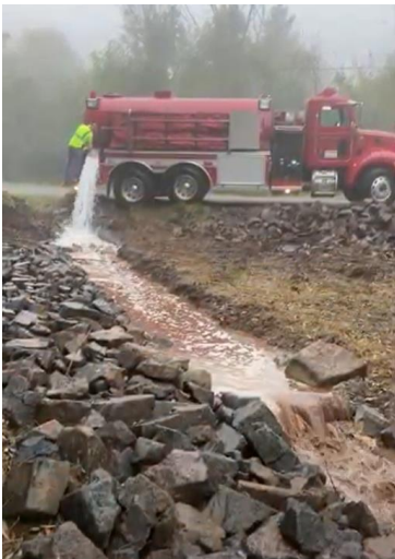
Flushing the new stream section to wash away sediment and get to a harder structure.
