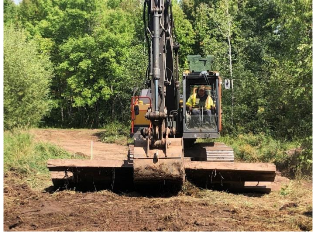
Laying timber matting for stream work in a wetland area.
