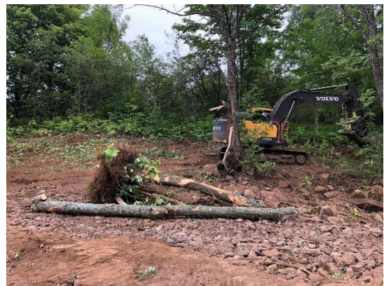
Harvesting material for the stream habitat construction.
