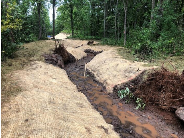
New stream channel completed, seeded, and erosion blanket installed.
