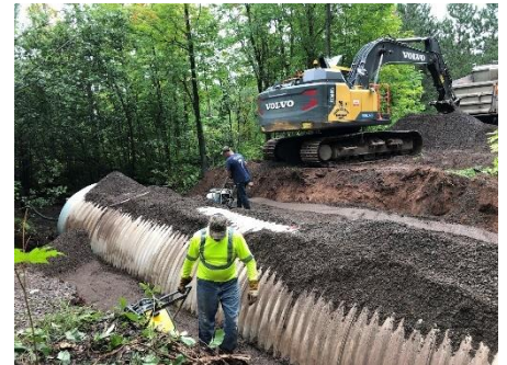
This project included 4 culvert replacements on town roads, 2 new culvert crossings on town roads, and 2 culvert replacements on private driveways where Kaari Creek flowed.
